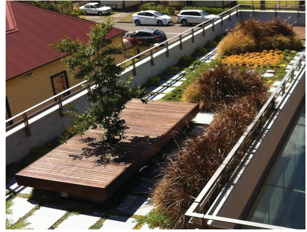
Photo 3: Green roof, Teralba. (Photo courtesy of Umwelt)
